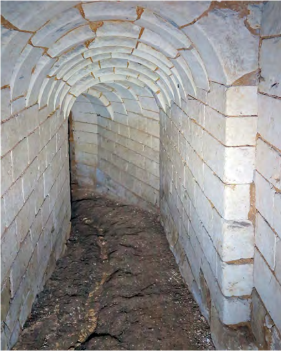
Entrance passage at Filescamps showing stepped ceiling of fine masonry
